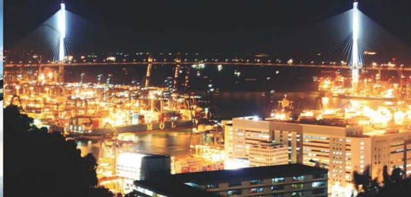
STONECUTTERS BRIDGE - HONG KONG
